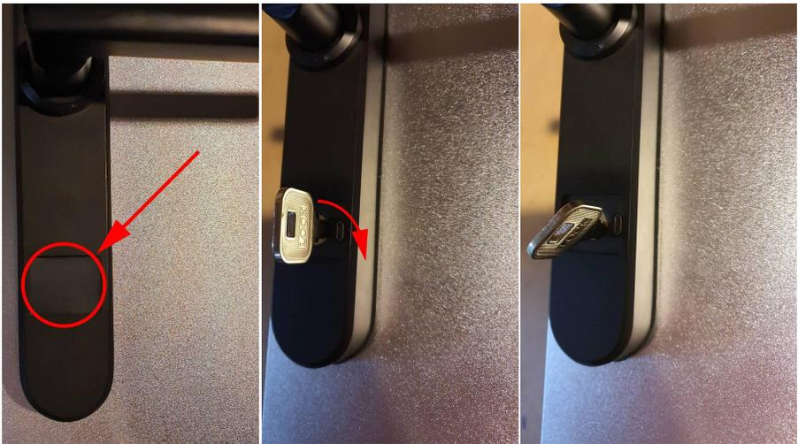
Shown on the right is the location of the mechanical key barrel, with cover removed.
